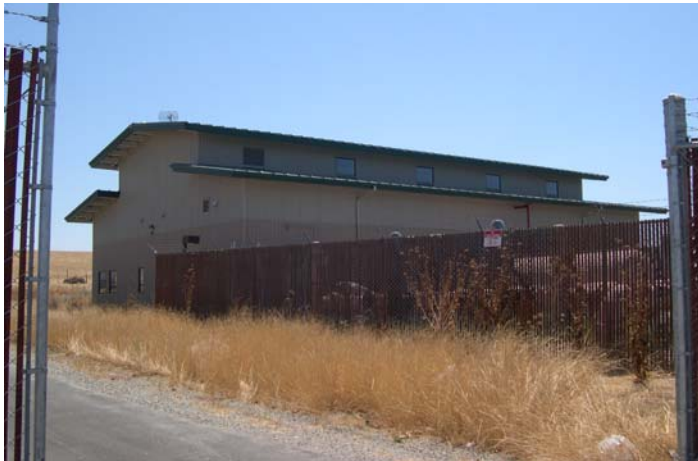
Photograph 2-1: Lessalt Water Treatment Plant
