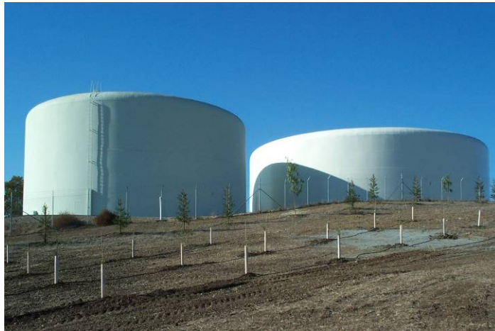
Photograph 2-2: Fairview Road Tanks
