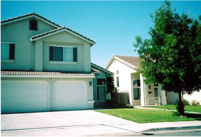
Photograph 1-2: High Mineral Content of Groundwater Impacts Residential Customers
