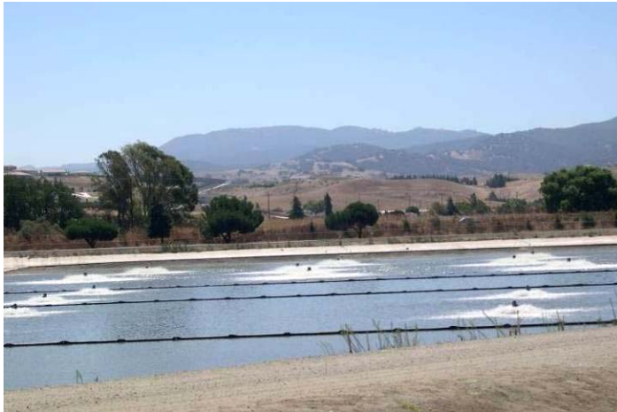
Photograph 3-1: Aeration at DWTP Pond
